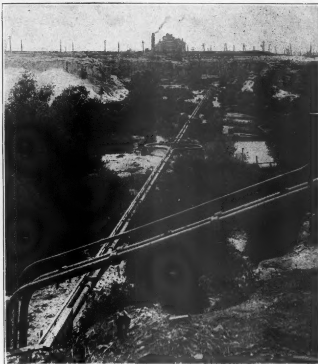
Steam Line to Plant B
